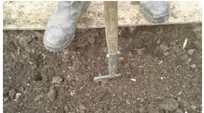
16 - Loosen the lower part of the trench another 30cm deep
